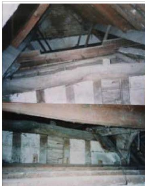
Timber-framed walls visible in roof-space
