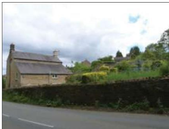
Rear of Hill House
