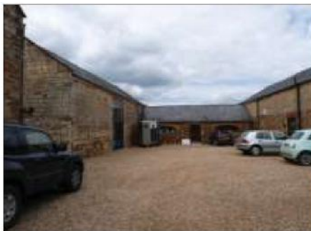
Wellington's converted farm buildings
