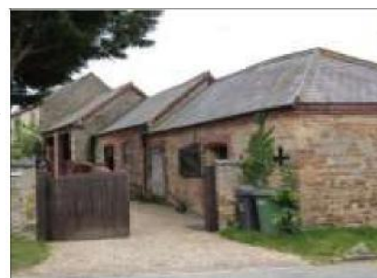
Stables at Woolpack Farm
