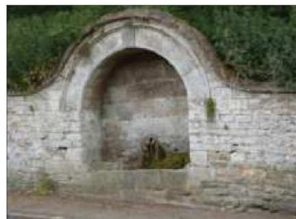
Water trough, The Hill
