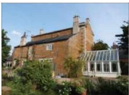
Rear range with lean-to roof
