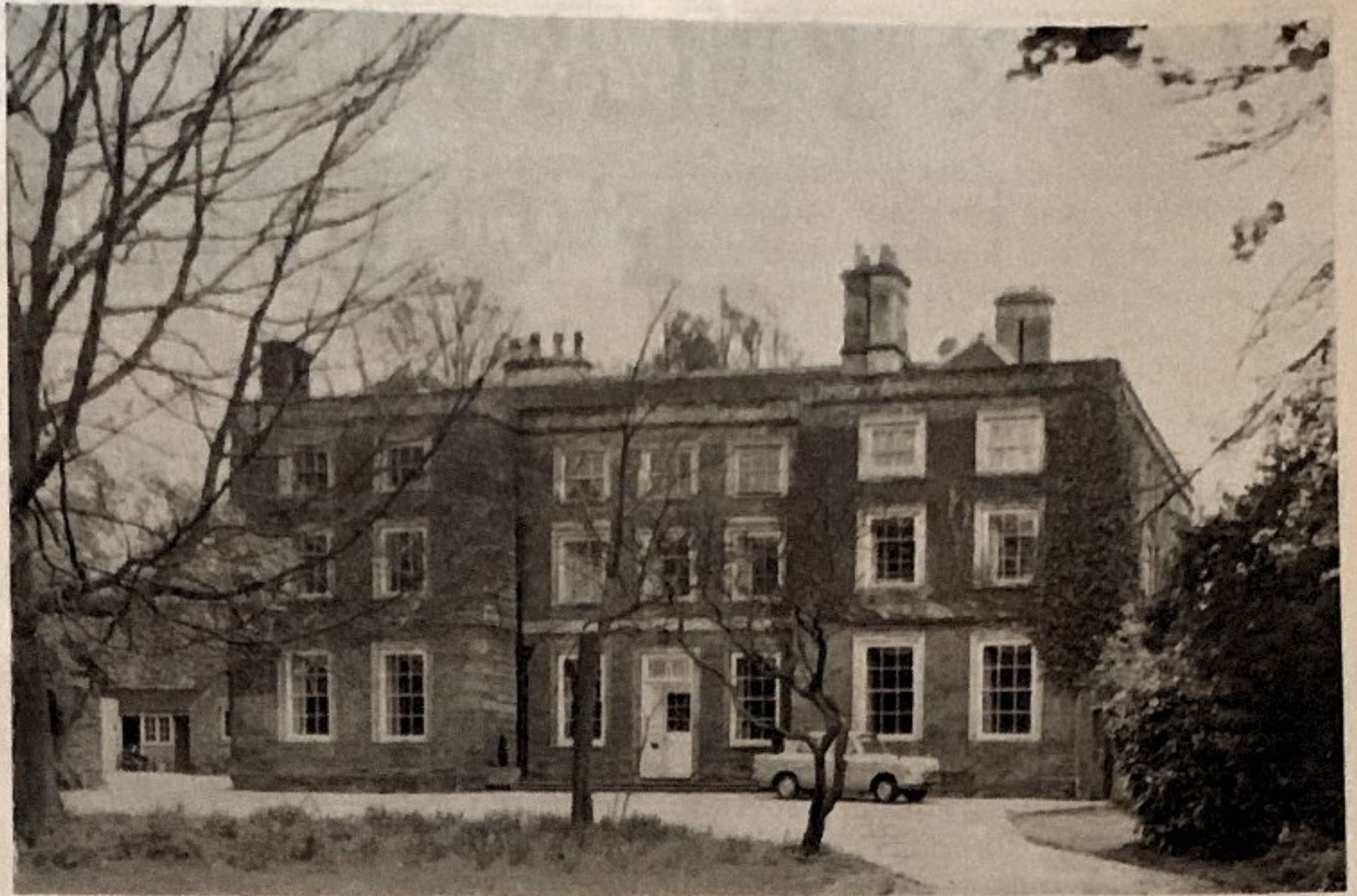
Bury House, Cottingham, one of the finest houses not only of the village but also of the County.
